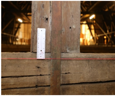
Figure 16 a)–c). Notable deviation from conventional engineering practice. The tie beams exhibit inverse deflection (left). Rather than maintaining a gap between the king post and tie beams, the beams are fitted with stirrups that induce upward tension toward the post (middle). Consequently, the entire truss assembly is tensioned, initiating at the tie beams and subsequently tightening each truss joint in progression.
