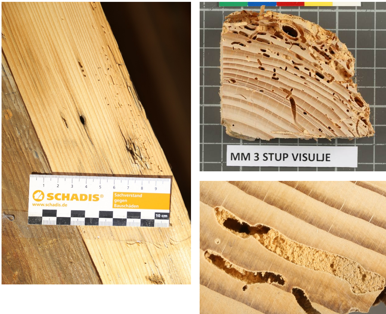
Figure 2. Left: half of the top surface of the beam was slightly planed to clean the dust and dirt. Damage can be seen only from sporadic exit holes, and only in sapwood-containing edges of the beam. Top right: polished cross-section of the edge of the beam containing a large amount of sapwood and larval tunnels. Bottom right: enlarged larval tunnel filled with coarse excrement.
