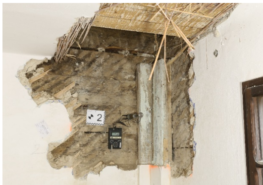
Figure 6 a)-c). Corner of the parish house in Mala Gorca (around 1830s). Initially, poor craftsmanship of the corners (dovetail notched joints) rendered the walls unstable. To address this, the walls were adequately, though not stylishly, improved by binding them with vertical planks and through the use of threaded bolts. Later, in the late 19th century, they were reinforced and plastered on both sides.
