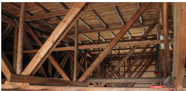
Figure 3. Measurement of the moisture content in roof timber trusses
