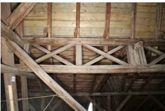
Figure 15 a) and b). At a span of 6.5 meters between the trusses, only a truss configuration is structurally feasible for the purlin. Minimal deflection is observed, while the roofing plane remains properly aligned. The precise assembly sequence of the complex joint is reflected in the firm and tight joints, demonstrating superior workmanship.
