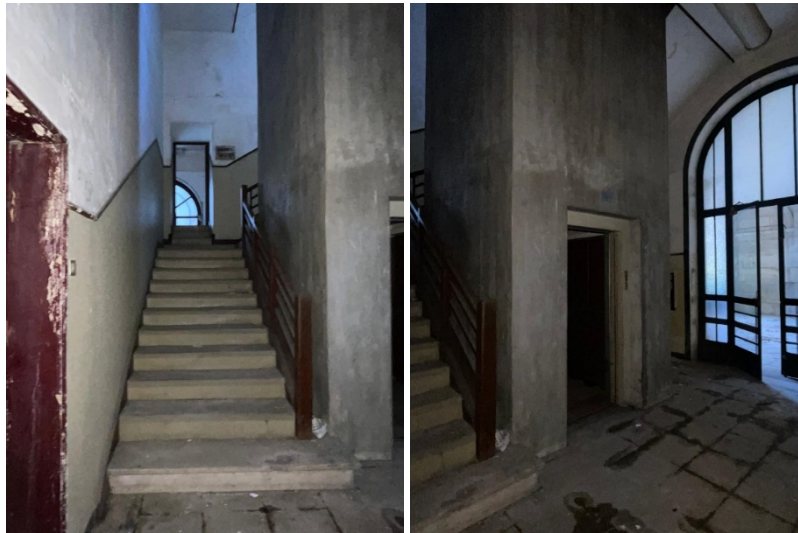
Figure 3. Reinforced concrete stairs and elevator shaft
