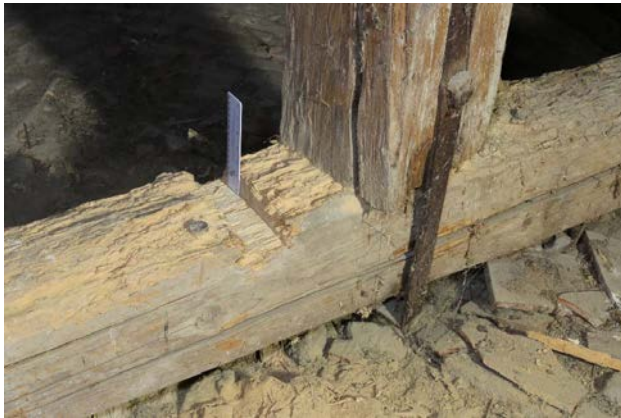
Figure 5. The tie beam was hewn from a small-diameter log; consequently, the large portion of the upper surface and corners contained sapwood, which was completely eaten by insects, leaving only 53% of the effective cross-section.
