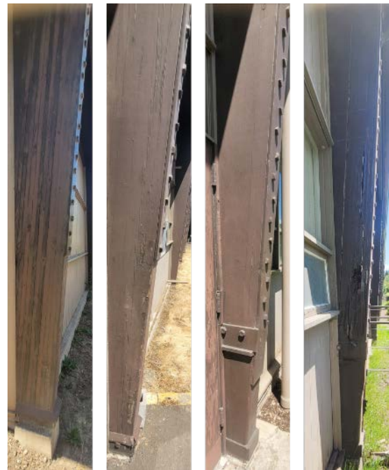
Figure 34. From left to right A13 with damaged coating, B8 with a wood prosthesis, D15 with a metal prosthesis and extended bracket, and D7 with notable brown rot in addition to a metal prosthesis and extended bracket.
