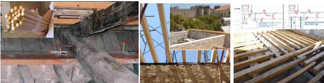
Figure 5: a) Hagi Mehmet Aga Mosque in Rhodes. a) Timber dowels ( d=14\text{mm} ) were used instead of steel dowels to connect the timber lacings to the masonry beneath, since steel dowels had often caused significant damage to the porous stones of Rhodes. Benizelos Mansion in Athens and the Turkish mansion in Rhodes [11]. b) In these cases, the usual cross timbers of the lacing system—normally placed above the longitudinal elements—were instead embedded within the masonry beneath the longitudinal timbers and connected to each other with screws ( d = 8\text{ mm} ) [8,12]. c) Timber floor beams screwed onto timber lacings anchored into masonry with stainless rods [11].
