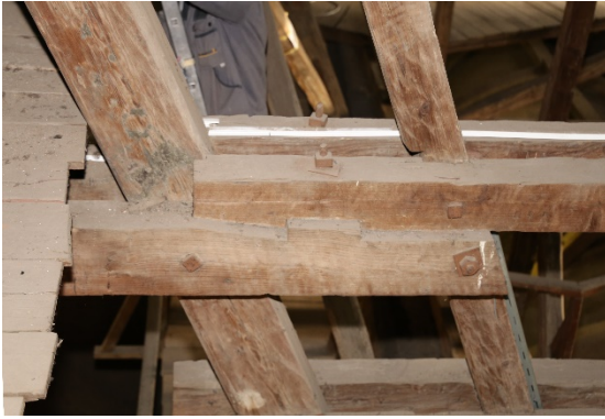
Figure 13 a) and b). Analysis of the joint between the principal rafter, double collars, and purlin to the side aisle. The crossed tenon lap joint between collars and rafter is very stable, with multiple half-lap joints secured by iron bolts. Interlocking in all three directions was assessed first. Subsequently, no wood failure—either in shear or in tension perpendicular to the grain—was recorded at any stage.
