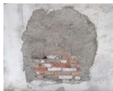
Photo 2 – 1 st and 2 nd floor wall
