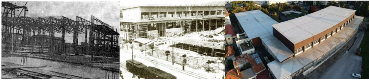
Figure 2. Photos from the construction phase of the museum AND museum building filmed by UAV
