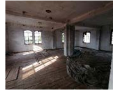
Photo 4 – Second floor of the extension
