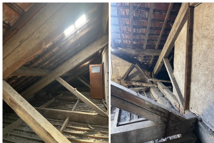
Figure 6. The roof structure is made out of wooden trusses with various geometries
