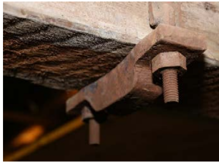
Figure 16 a)–c). Notable deviation from conventional engineering practice. The tie beams exhibit inverse deflection (left). Rather than maintaining a gap between the king post and tie beams, the beams are fitted with stirrups that induce upward tension toward the post (middle). Consequently, the entire truss assembly is tensioned, initiating at the tie beams and subsequently tightening each truss joint in progression.
