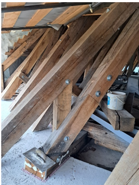
Figure 8 a) – f). Church of the Ascension of the Blessed Virgin Mary in Pokupsko (late 1700s). The Oakwood structure was damaged by distortion and opening of the joints and by biological damage (upper left). A reinforced concrete ring girder replaced wall plates, and rotten elements were partly replaced with prostheses. Tie beams and struts are now insulated in the concrete; the sprockets with birdmouth joint sit on the end of the beams (end grain opened for drying). Tenons and stop-splayed scarf joints with keys or wedges were used in reconstruction. These joints are fixed with threaded rods instead of the original wood pegs for reasons of better tightening and strength. Right column: Experts' sketches for the execution of joints and discussions with carpenters.
