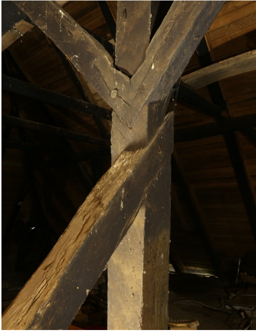
Figure 5 a) and b). Dovetail lap joints have too small an angle ( <10^\circ ). When positioning two adjoining dovetail laps, poor alignment can cause wedge-like action, resulting in splitting of the post. To address this issue, refer to the suggested joint for this purpose located at the lower right.
