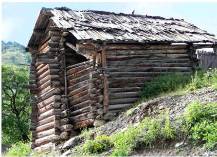
Figure 13. A log building from Günpınar village (Photo: Küçükbaş, A.)
