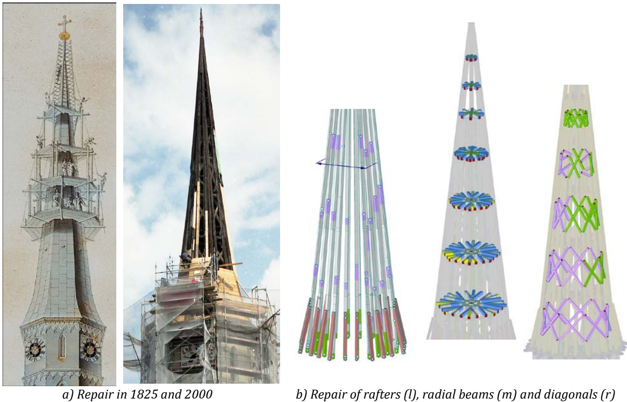
Figure 5. Numerous repairs over centuries
