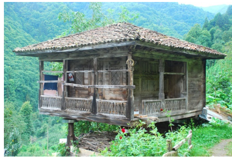
Figure 14. A block building from Rize (Photo: Dışkaya, N.)
