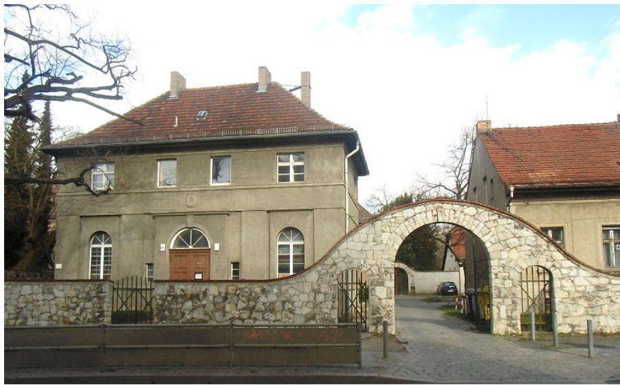
Figure 6. Exterior view of the Margarethenhaus, Berlin, before the extensive redevelopment
