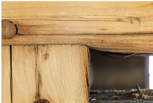
Figure 7 a)-c). Structure above the side aisle of the Zagreb Cathedral (1898). Each of the four segments of the roof with side gable walls spans approximately 6 m. To address this span, the solution involved constructing a beam-like structure, featuring wooden beams as flanges and wooden blocks with through bolts as a web (see lower detail). However, the structure deflected, partly due to the drying of the wood and the pressing of bolt washers into soft firwood, and partly due to the eccentricity of the loading. Additionally, the minimal end-grain surfaces of the queen posts caused compression crushing perpendicular to the fibres of the collar beam (left).
