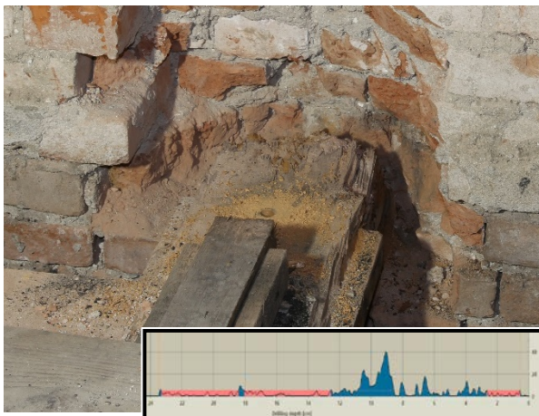
Figure 3. Regular problems with the wood beam inserts in the wall. Photographs: whenever the beam is built in tightly, with no insulation or ventilation, total damage occurs. The sketch represents the optimal firm insert of the beam into the wall, insulated from moisture at least from below, and ventilated by alternate shifting of bricks at the end grain and the sides.
