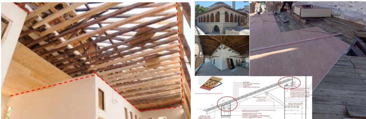
Figure 3: a) Benizelos mansion in Athens. Application of 20mm plywood over the ceiling, with both layers screwed onto the ceiling beams of the roof (horizontal plane) [8]. b) Kaloutsiani Mosque in Ioannina. Application of plywood over the interior visible timber planks. The inclined timber diaphragm, anchored to the masonry walls through timber-tie beams (red circles), was used to enhance the seismic resistance of the angular porch, especially against out-of-plane forces [9].
